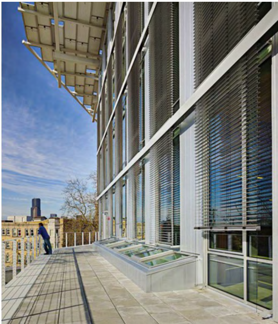
Figure 29. South terrace at level 3 showing exterior blinds deployed and tilted for maximum daylight.
