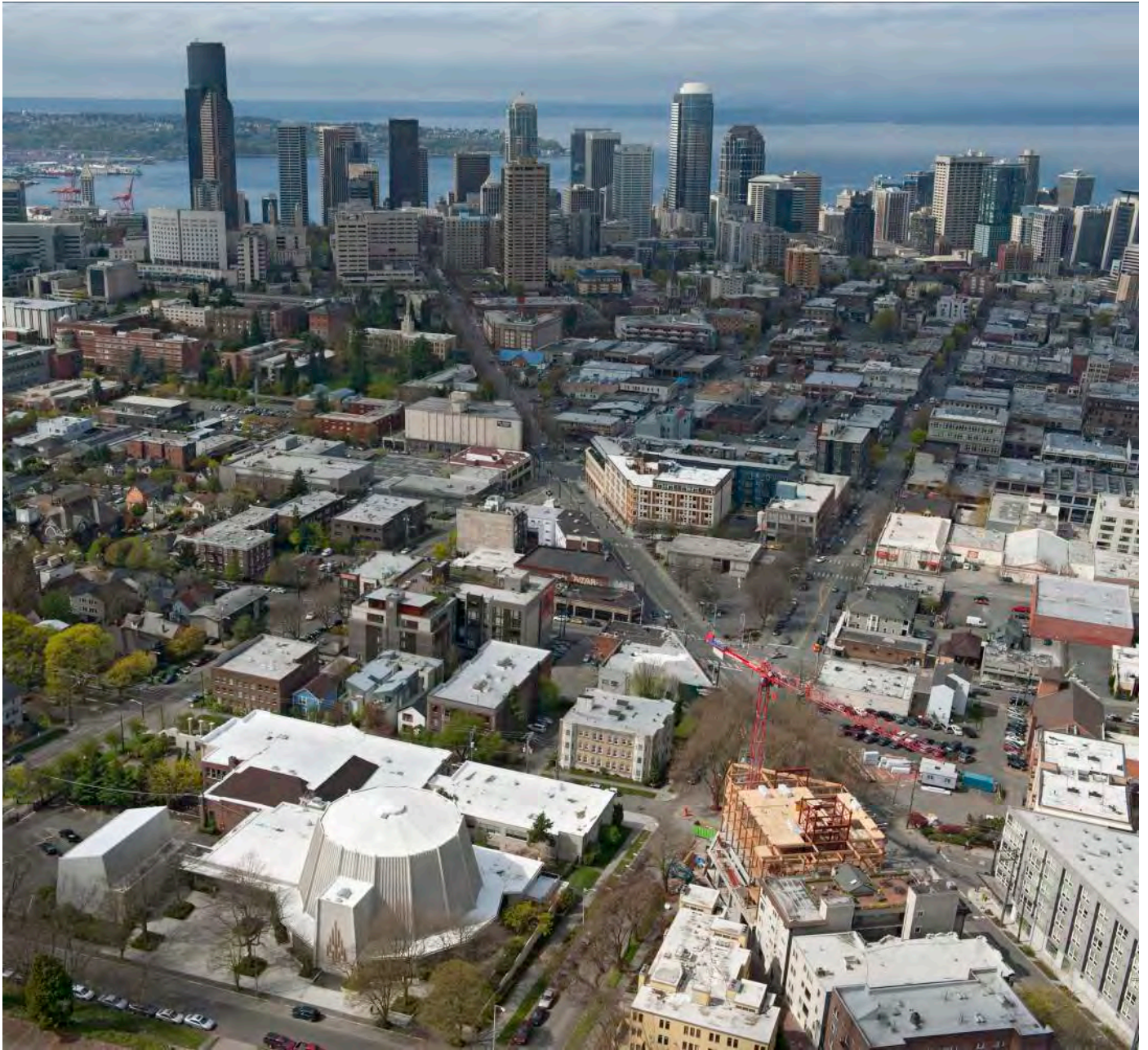
Figure 8. Aerial view of the Bullitt Center under construction, spring 2012 (John Stamets)
